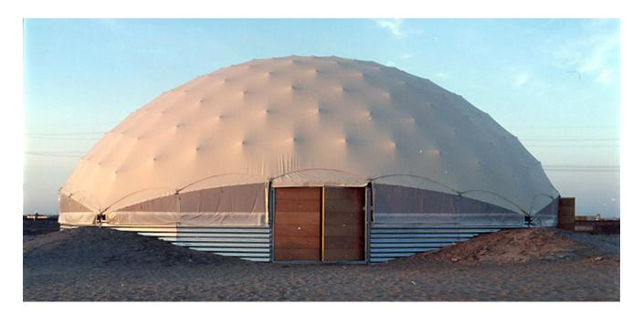
The Nomadic Paper Dome is a hemispherical paper tube structure designed as a temporary theater for a mime group in Amsterdam. The choice for the specific materials and structure - a grid of short paper tubes held together by star shaped joints - had been determined by the temporary character of the building. The demand for easy disassembly and re-assembly, and the wish to use only affordable and re-usable materials were also taken into consideration.
