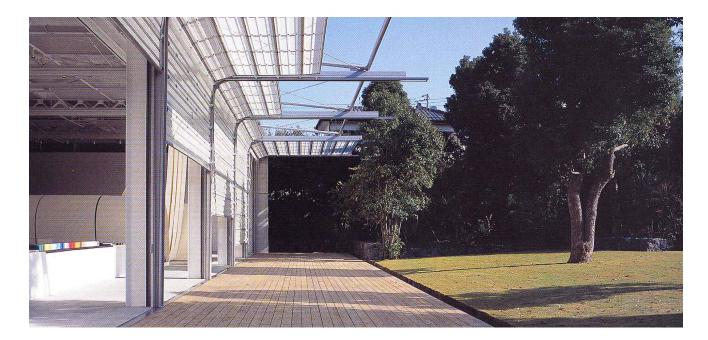
For the 924-square-meter contemporary gallery, an existing structure was renovated. A similar transformation occurs on its south facade. This entire side is composed of six sets of translucent fiberglass-reinforced plastic (FRP) shutters that look like shoji screens when closed. The panels slide outward, creating a 5-meter-deep awning, and the interior gallery extends outside and reconnects with the surrounding landscape.
