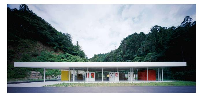
The main design focus for this children's art museum was to create an ideal facility made of a material familiar to children, where they could exhibit their art work in purely natural light. The triangular roof is made of paperhoneycomb arranged as equilateral triangles, connected by only three different simple joints. The paper structure is covered with corrugated plastic, which is then finished with a PVC membrane, allowing natural light to uniformly penetrate through the whole structure.
