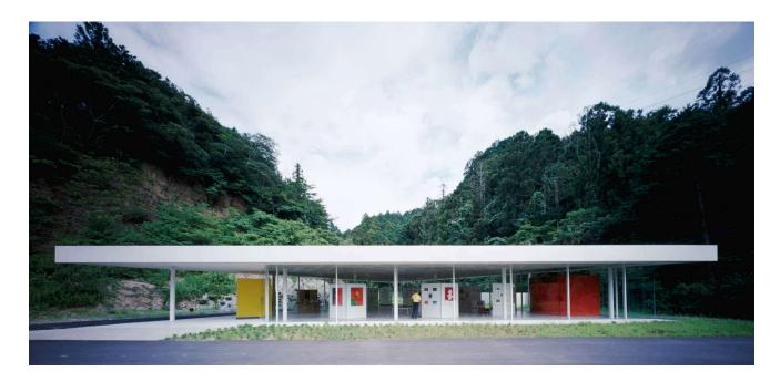
The main design focus for this children's art museum was to create an ideal facility made of a material familiar to children, where they could exhibit their art work in purely natural light. The triangular roof is made of paperhoneycomb arranged as equilateral triangles, connected by only three different simple joints. The paper structure is covered with corrugated plastic, which is then finished with a PVC membrane, allowing natural light to uniformly penetrate through the whole structure.
