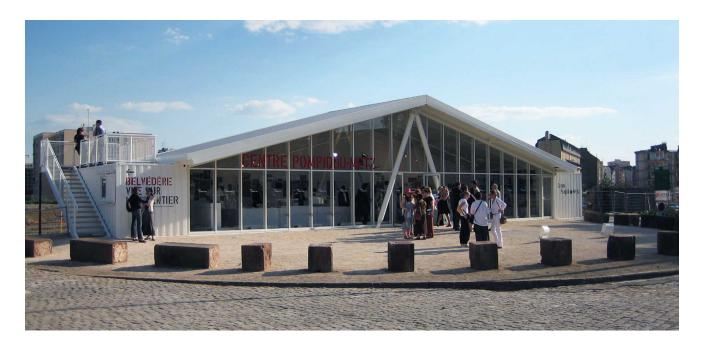
To inform the inhabitants and visitors of Metz about the design and building process of the new Centre Pompidou Metz, a temporary exhibition space was built on the site. The main structure consists of a light corrugated steel roof spanning between two rented containers. The containers function as structure and storage space and at the same time can be used as a belvedere on the building site.
