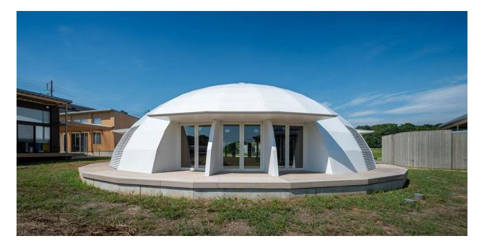
This dome is a part of Keio University's SBC project (Student-Build Campus). Since the construction work by students was required, we used a PHP panel with a honeycomb board as the core material, so that the frame was kept to a weight that enables the student to carry. PHP panels are gathered in a central ring to form a 14m diameter pillarless space.
