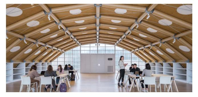
This dome is a part of Keio University's SBC project (Student-Build Campus). Since the construction work by students was required, we used a PHP panel with a honeycomb board as the core material, so that the frame was kept to a weight that enables the student to carry. PHP panels are gathered in a central ring to form a 14m diameter pillarless space.
