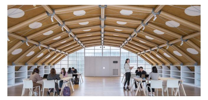
This dome is a part of Keio University's SBC project (Student-Build Campus). Since the construction work by students was required, we used a PHP panel with a honeycomb board as the core material, so that the frame was kept to a weight that enables the student to carry. PHP panels are gathered in a central ring to form a 14m diameter pillarless space.
