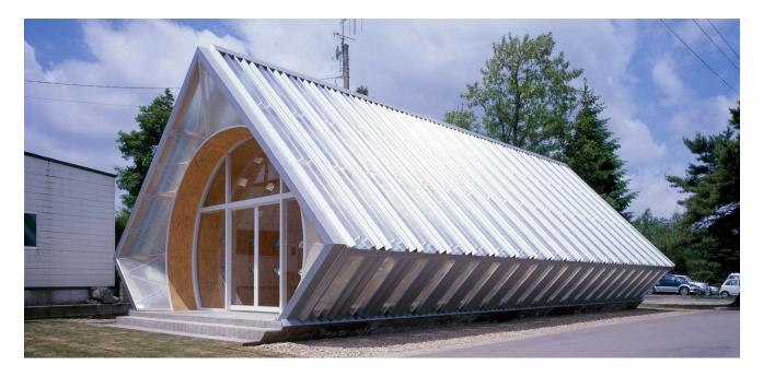
The main space of the Daycare Center is created with LVL wood, the same as the roof material of the Uno Chiyo Museum. Because the shape of the tunnel arch puts the members in compression, the thickness of the veneer needed to be increased, which made it impossible to weave. Instead, the grid-shell was created by bending and bolting the members. A secondary roof with a 45 degree pitch was created for snowfall, insulation, and stability.
