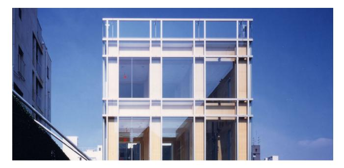
The building's structure is made of one-story-high Vierendeel trusses spanning 22 meters on every other floor, allowing open spaces for showrooms, offices, and meeting rooms. The way structural timber members can be thickened for fireproofing, this steel structure is covered by wood, functioning as finishing and fireproofing at the same time, therefore minimizing costs and resources.
