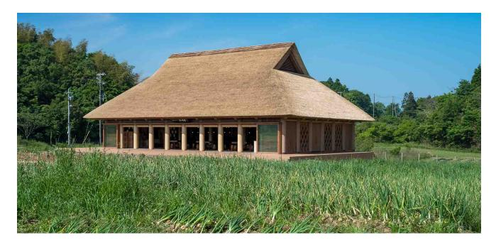
The restaurant is built in the midst of a large natural field and serves fresh vegetables from there. The thatched roof used in traditional Japanese farmhouses and the large roof assembly made of a hybrid structure of paper tubes and wood create a spacious area with high ceilings, which is also used as a music hall.
