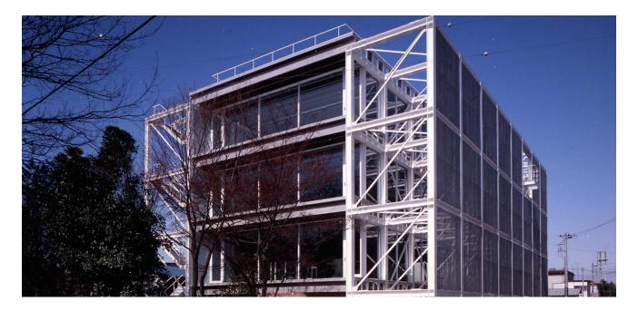
Budget constraints, a tight schedule, and the requirement to accommodate heavy machinery yielded a design with pre-cast, pre-stressed concrete slabs pin-connected to two four-story steel frame structures taking all horizontal loads. With no beams or bracing spanning between the two steel structures, the slabs could be easily craned in to position. Furthermore, the factory's machines could be inserted without interference.
