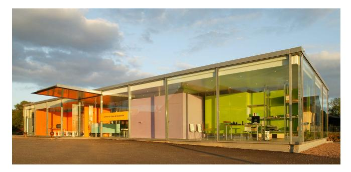
Conceptually parallel to the Furniture House, this gallery space contains a series of exhibition units that double as structure. Each unit is made of readily available perforated steel shelf angles, which are used throughout the building for a wide range of functions such as display units, storage cabinets, and wall partitions.
