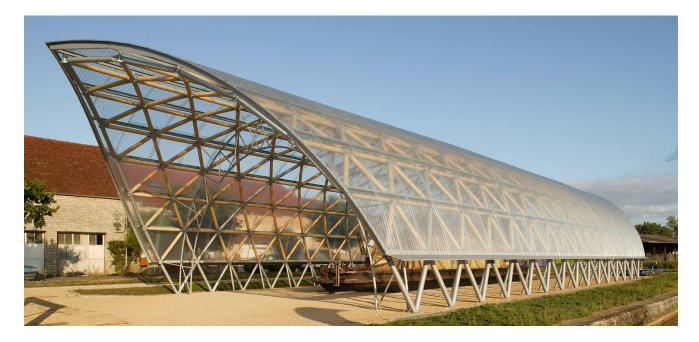
This boathouse, sheltering a historically significant canal boat, is made of a triangular-lattice paper-tube grid-shell structure, covered by corrugated polycarbonate panels. Die-cast aluminum joints were developed in order to use the same-sized paper tubes and testing data of the Japan Pavilion in Hannover for approval in France.
