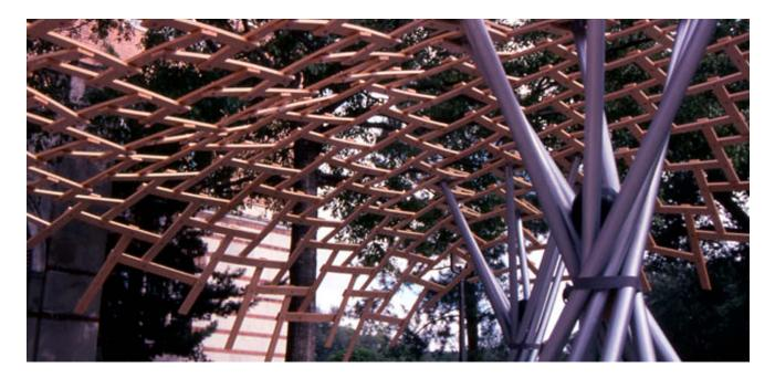
A half-scale prototype of the "Forest Park Pavilion" in St. Louis, the Bamboo Roof is comprised of groups of four boards that are overlapped in a spiraling pin-wheel connection. Different orientations of the overlap result in a change in curvature. This arrangement of pin-wheel connections creates a pattern of large and small squares, and forms a concave or convex geometry resulting in a shell structure or grid shell.
