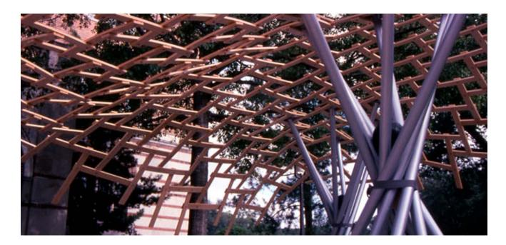
A half-scale prototype of the "Forest Park Pavilion" in St. Louis, the Bamboo Roof is comprised of groups of four boards that are overlapped in a spiraling pin-wheel connection. Different orientations of the overlap result in a change in curvature. This arrangement of pin-wheel connections creates a pattern of large and small squares, and forms a concave or convex geometry resulting in a shell structure or grid shell.
