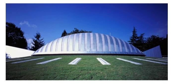
As an initial response to the small buildings surrounding the site, which include houses as well as a kindergarten and hospital, the bulk of the gymnasium was placed underground. A developed version of the Imai Daycare Center, the structure of this dome was a lattice of laminated strand lumber (LSL). Trussed arches spanned the short axis and parallel Vierendeel arches crossed the major axis.
