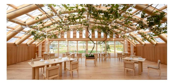
This greenhouse is composed of arches made from paper tubes connected by metal joints. on the exterior, a ready-made greenhouse frame was installed with a double layer of fluorine film with an air layer in between to suppress the temperature changes of the interior. In summer, the leaves of the plants grown inside will cover the ceiling, blocking sunlight.
