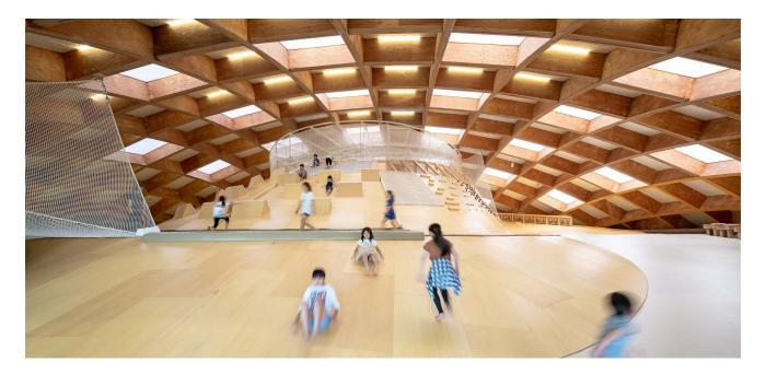
In developing a dome with a diameter of 35.6m and a height of 6.95m, the idea was to use an inexpensive and light-weighted box beam (PHP system) of paper honeycomb board sandwiched in structural plywood, as a substitute for huge glulam arches. However, with a large span and snow load, the paper honeycomb was replaced with a regular wooden box beam. The next project, Student Built Campus at Keio University SFC implemented the PHP system.
