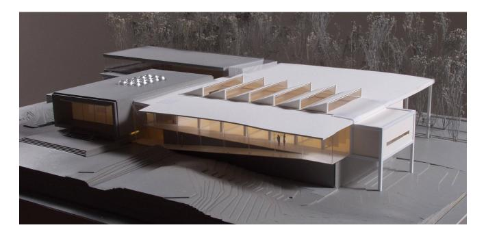
The design for the renovation and expansion of the Rose Art Museum strives to integrate the new and renovated programs economically, functionally, and aesthetically within its context. A Vierendeel truss supports the roof over the main exhibition space allowing for a flexible gallery as well as a large glass facade which connects the main exhibition space to the activity of the surrounding Brandeis University campus.
