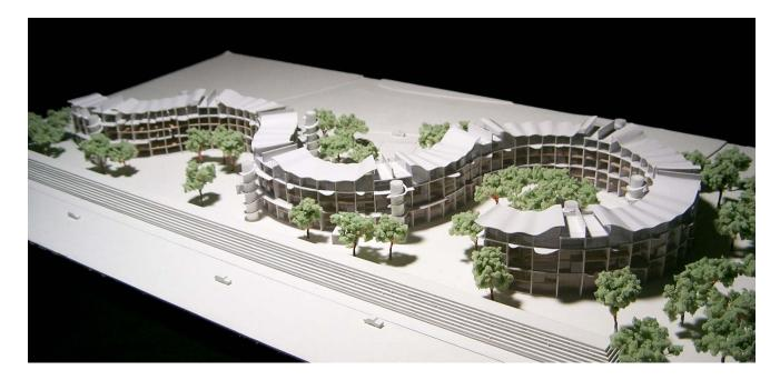
The apartments planned for Bong Mu in South Korea are free of transversal walls, allowing for cross-ventilation and openness. The overall structural system is achieved by transferring lateral forces through floor slabs from one wall to the next, the S-shape of the building gives balance to the structure.
